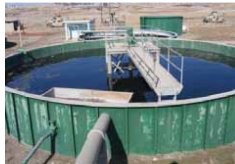
A view of the Kirkuk Al Rashid Wastewater Treatment Plant.
